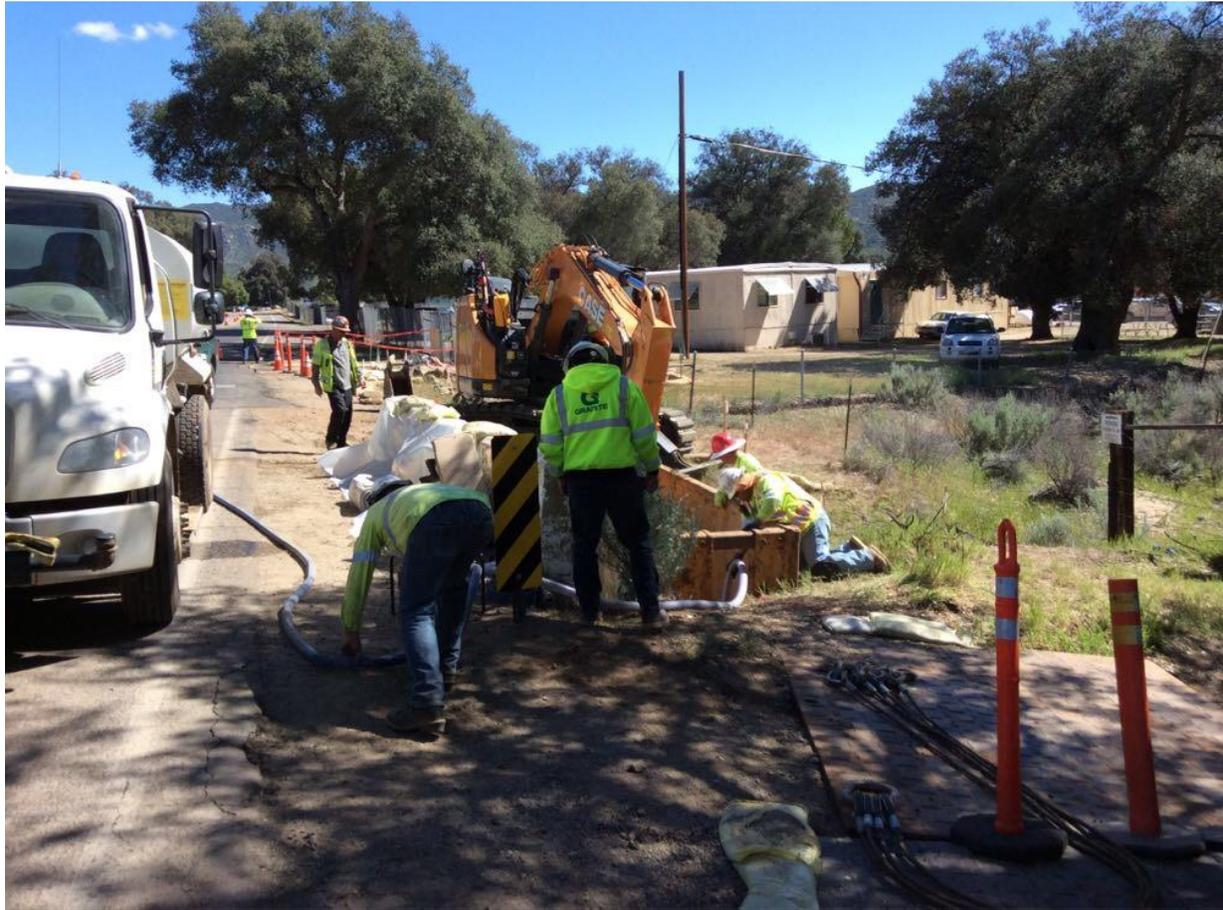
**Photo 4:** Groundwater encountered in the ephemeral stream channel near 19+96 was pumped into a water truck and later dispersed onto Morena Stokes Road on C 449 in accordance with APM HYD-08 and MM BIO-1.
