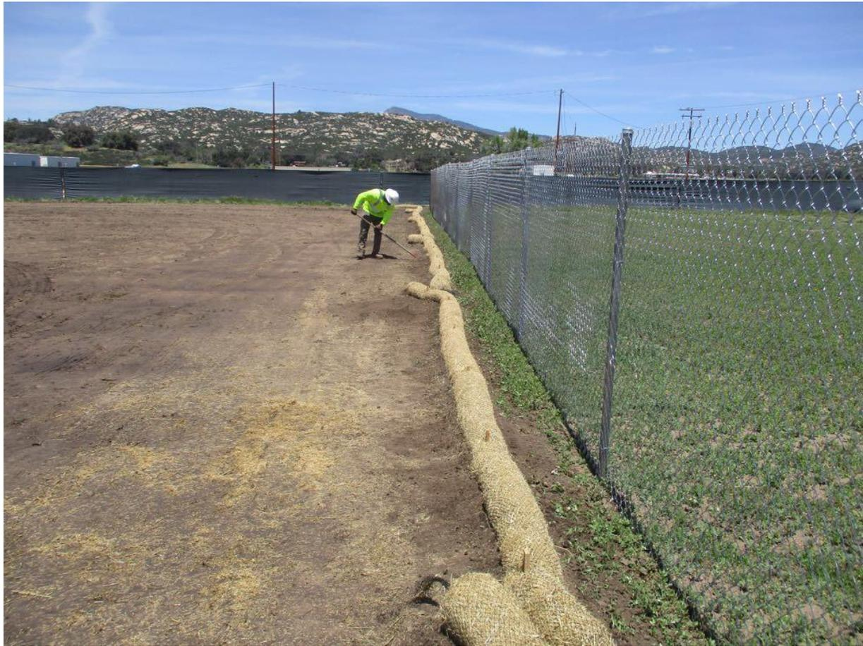
**Photo 2:** A crew member was observed finishing the installation of BMPs (straw wattles) along the perimeter of Merrigan Staging Yard expansion on TL 629A in accordance with the Erosion Control Plan and SWPPP. Opaque visual screening fencing was observed installed at the Merrigan Staging Yard (TL 629A) in accordance with APM VIS-02.
