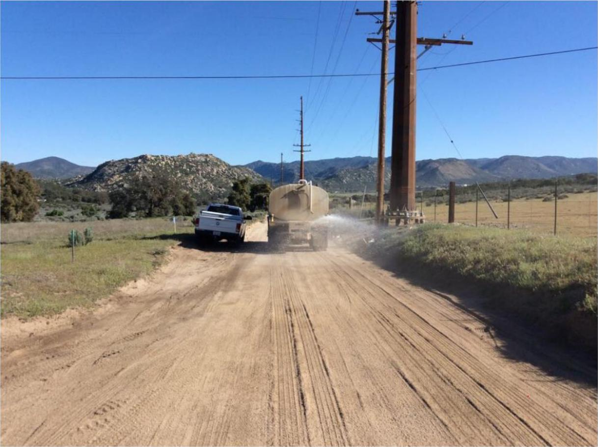
**Photo 5:** A water tender was observed applying water to the access road along TL 6958 to minimize dust emissions in accordance with APM AIR-02.
