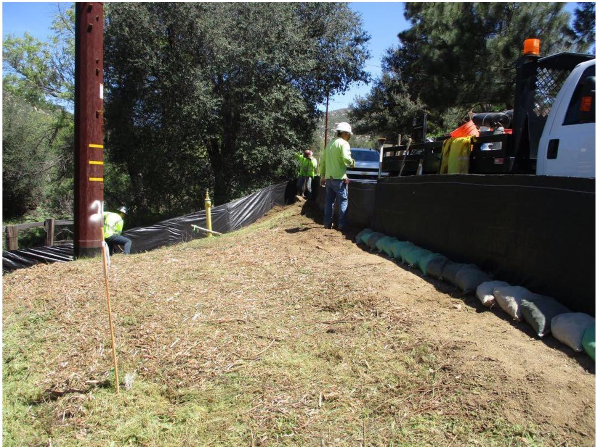
**Photo 1:** A construction crew was observed installing silt fence at Pole Z172800 (TL 629A) in accordance with the Erosion Control Plan (MM HYD-1) and was installed under the supervision of the Authorized Biologist per the recommended impact avoidance and minimization measures for the line.
