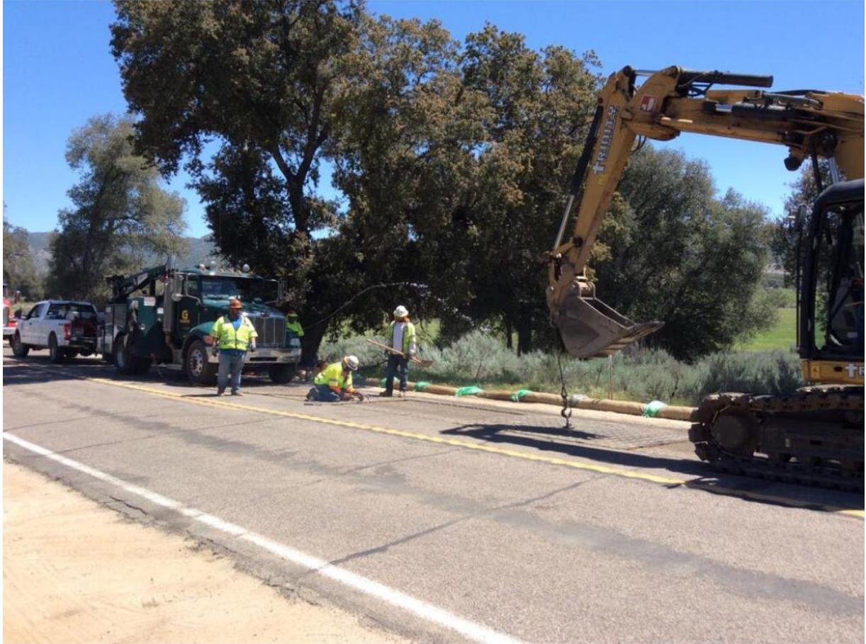
**Photo 3:** A dedicated fire patrol was observed wetting down the area surrounding hot work near along C449 and a complete set of fire tools was staged on site (5-gallon backpack pump, round point shovel, Pulaski, and 2A10BC fire extinguisher) in accordance with the CFPPP (MM FF-1).
